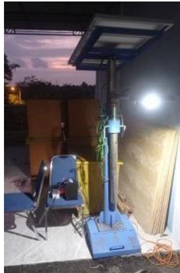
Figure 8. Experiment battery monitoring device at renewable energy laboratory
